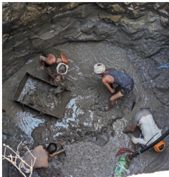
Well Construction Works in City
